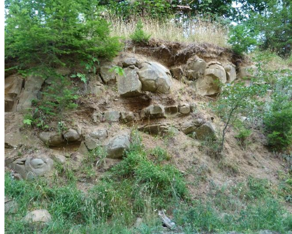
Photo 12. Cut through ridge with sandstone blocks and flaking mudstone.
